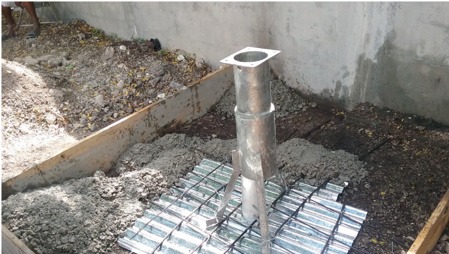
One more new pump being installed
