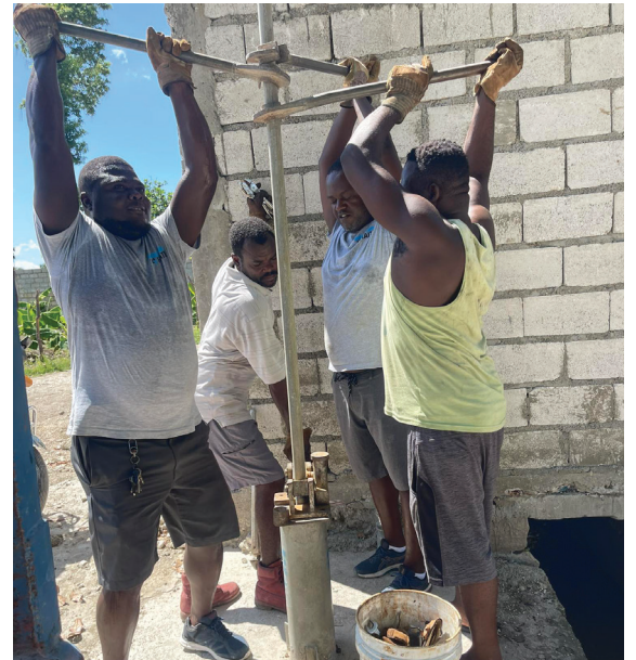
Repaired nearly 3000 pumps in 15 years
