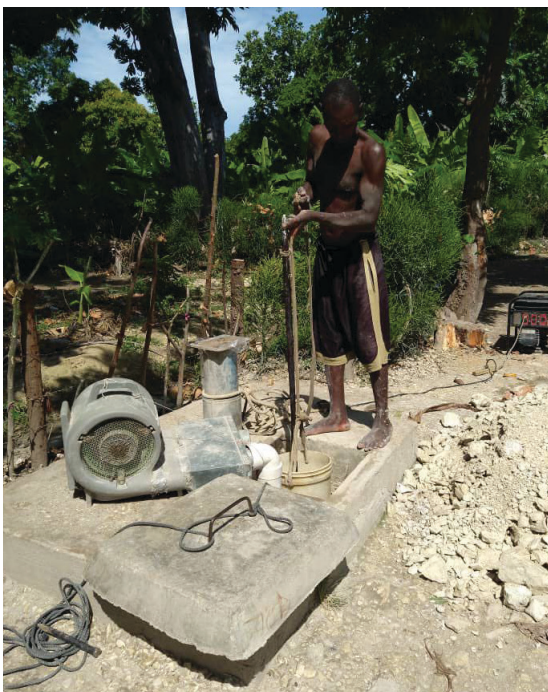
A fan set up to blow air to the digger
