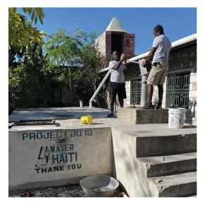
One of our first major projects years ago was the installation of this 25,000 gal cistern. It is 6' in the ground and 4' above. Water from a church and a school's roof is piped into the cistern. During the dry season we have to deliver water as the village has only salty water in the area. The pump is naturally only 10' deep but it works just like
