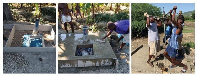
During our years in operation we have also dug close to 70 new wells. The photo shows a form around a pump set on a piece of tin covering a 30" hand dug hole to water. The small sq. form will allow access to the well in later years for cleaning. After the concrete has been poured, a few days later the crew will return and install the cylinder, pipe and pump assembly, lowering the pump through the stand and a 4' piece of pvc pipe through the tin down into the water.
