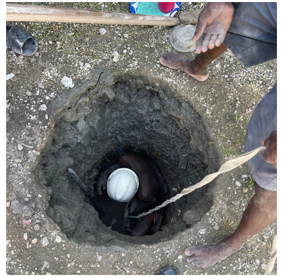
Yes, a man digging a 30" hole, going even to 90' to find water
