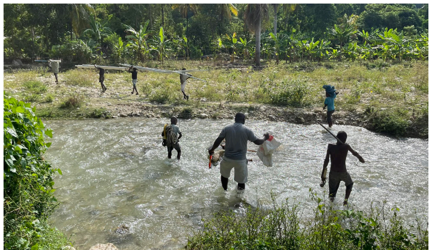
The broken pump is across the river, so carry everything needed
