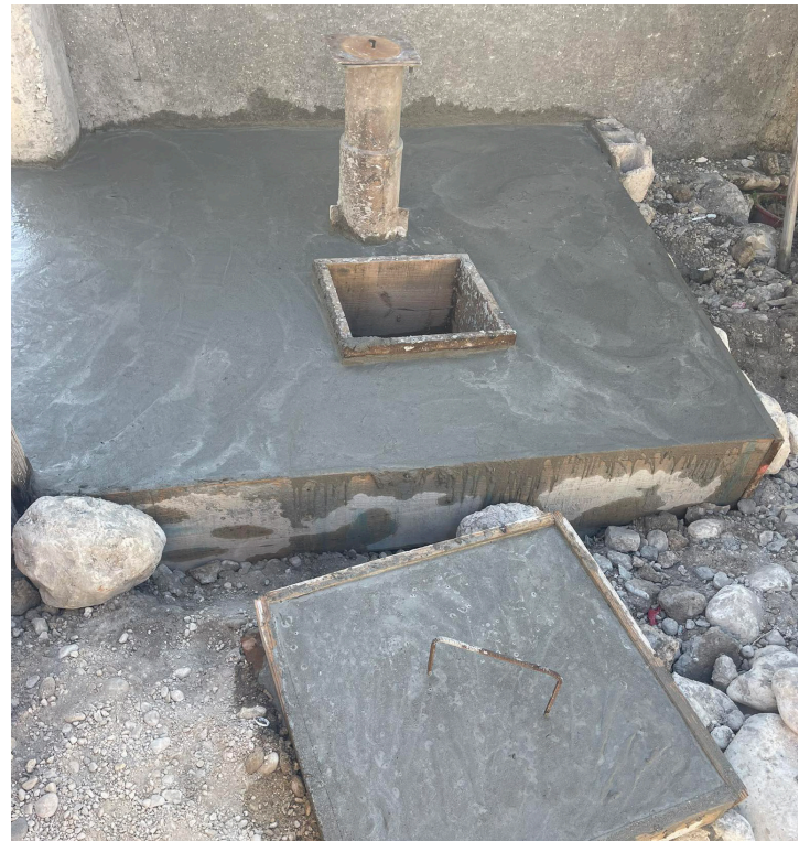
A finished pour of a pump stand and manhole lid
